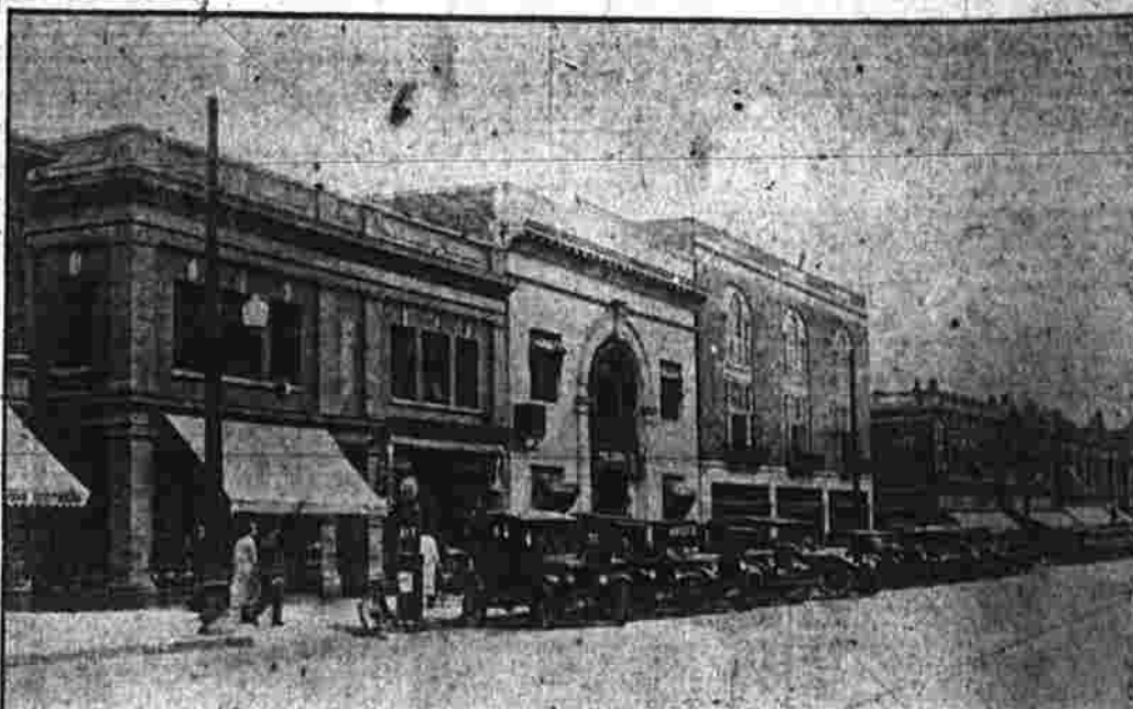
VIEW OF MAIN STREET LOOKING SOUTH.
